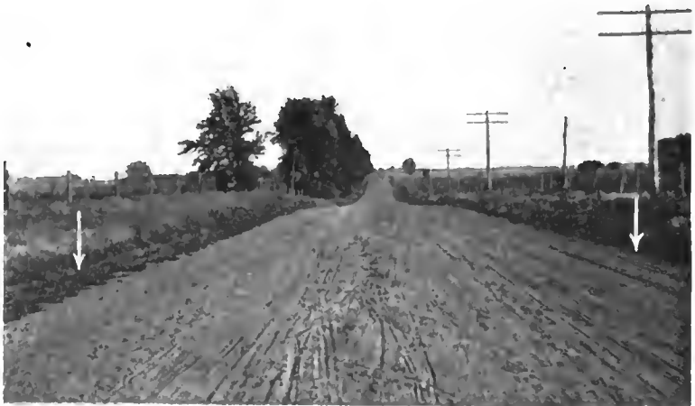
A gumbo road just commencing to dry out two days after a rain. On the extreme right and left are deep side drains, but the lack of crowning prevented the water from running off as it fell, making heavy going in the meantime. The right hand side is yet miry. Travel on the left has squeezed out most of the moisture, at the same time forming deep ruts to hold the next rain. Travel will then keep to the right which has become sunbaked in the meantime. And so it goes.
